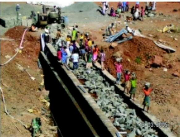
Work in progress on the bund
